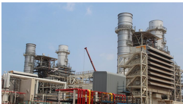
The 350 MW Kpone Independent Power Plant is among the largest independent power producers in Ghana. Photo by Cenpower.
