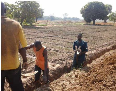
A watering system is under construction on the Diguissème rehabilitated site.
