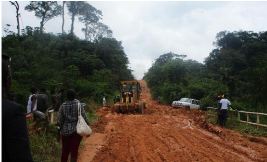
Road maintenance on the road to Sanniquellie, Nimba County's Capital
