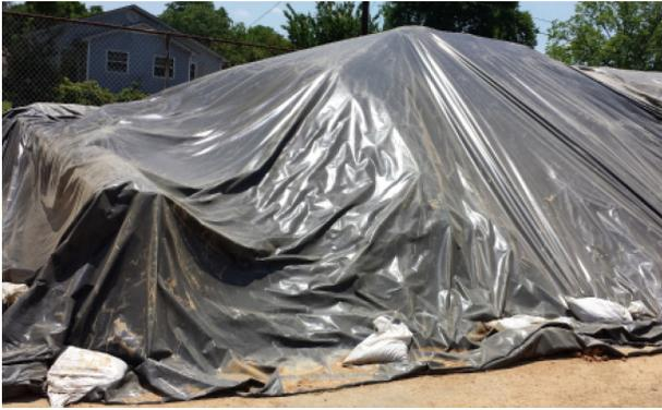
*Soil stored on site is covered with a tarp to prevent dust from blowing.*
