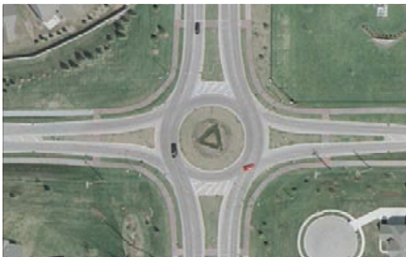
Figure 3 – Radial Design with vehicle entry path overlap problems addressed with improved striping. (Note: Non-radial design techniques used by Tetra Tech eliminate this problem with proper geometric and design vehicle considerations.)
