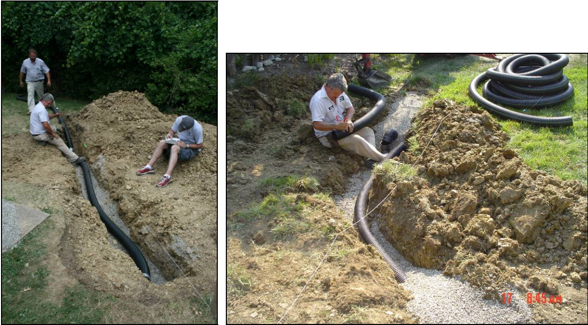
Figure 4 – Photograph of rain garden installation – underdrain installation
