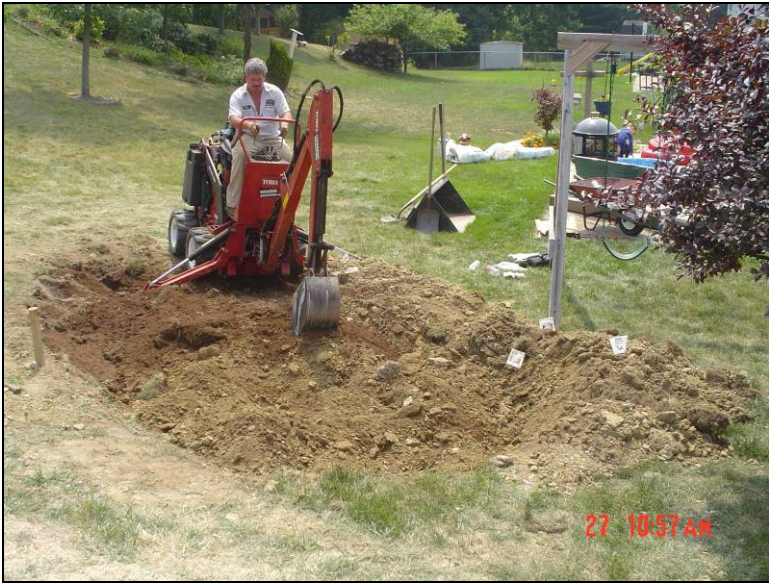
Figure 5 – Photograph of rain garden installation – mixing in soil amendments
