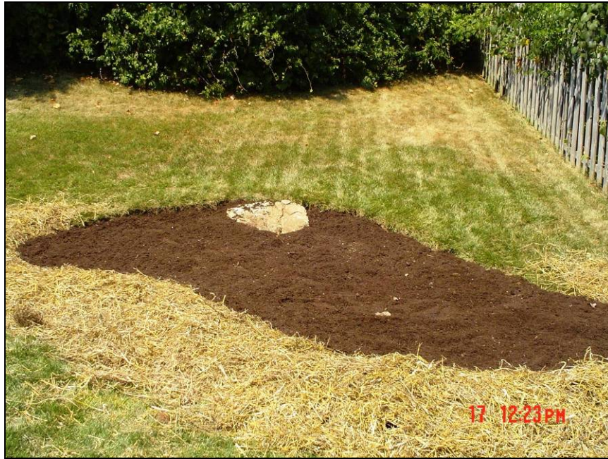
Figure 6 – Completed rain garden before planting
