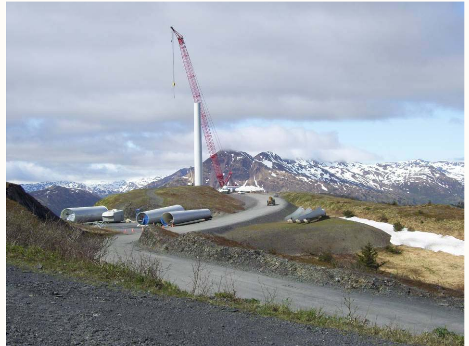
Construction of Kodiak Electric Association Pillar Mountain Wind Project
