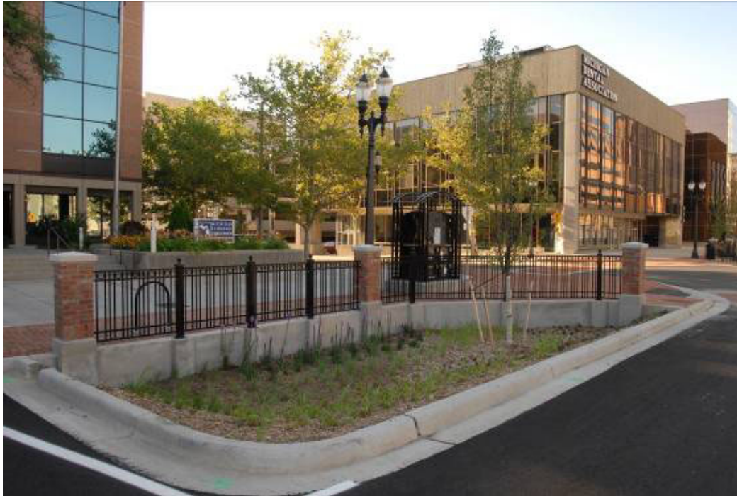
Urban Rain Garden, Washington Avenue, Lansing, Michigan Photo by Tetra Tech
