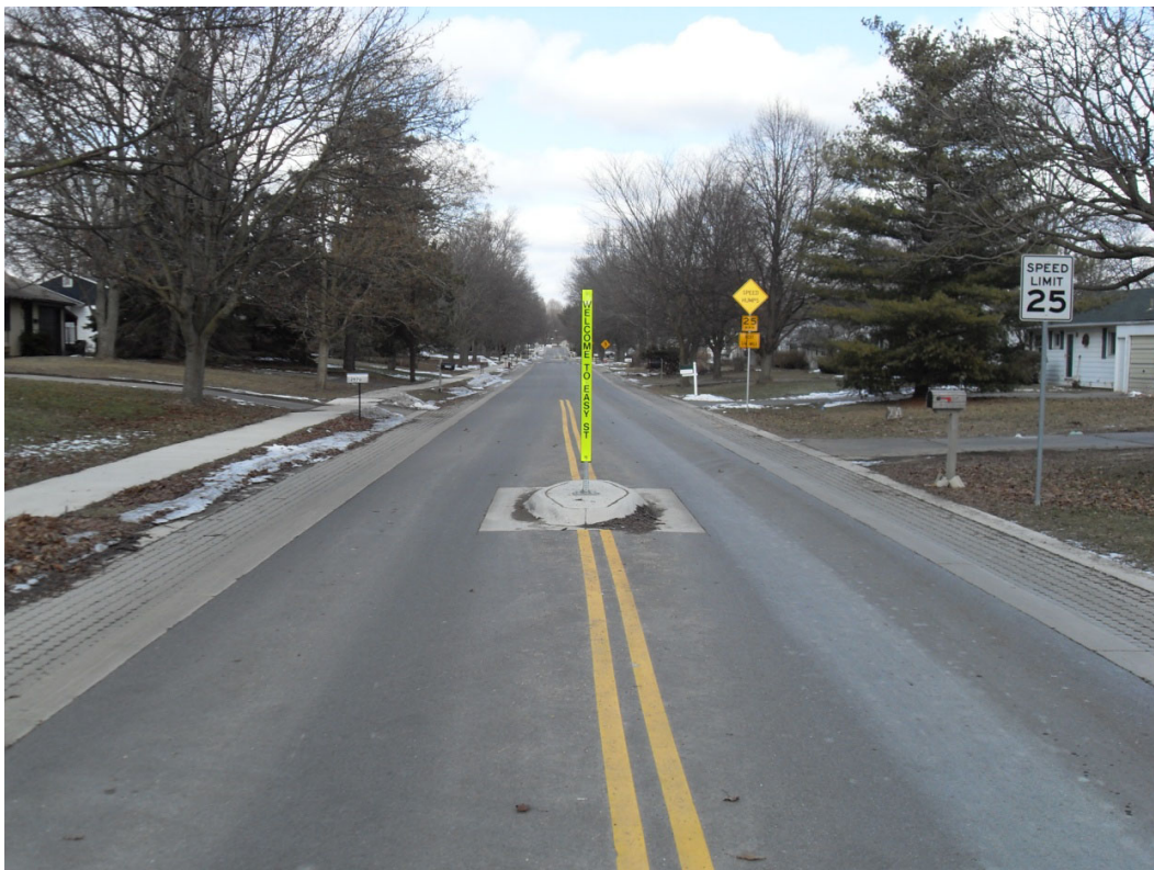
Easy Street, Ann Arbor, Michigan Showing Roadside Permeable Pavers and Swales Photo by Tetra Tech
