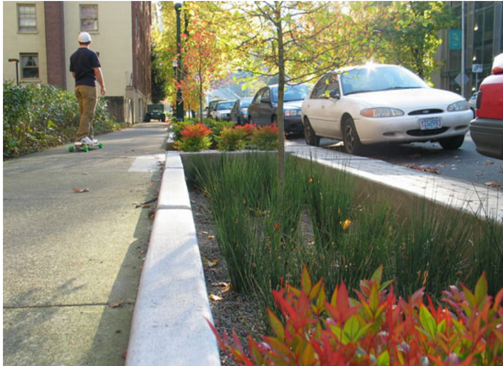
SW 12th Avenue Green Street Project, Portland, Oregon Photo by Kevin Robert Perry, City of Portland Environmental Services
