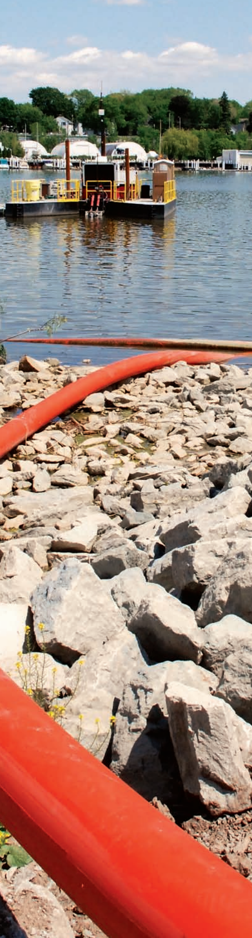
▲ Cleanup Crew. Clockwise from top, Tetra Tech's Ray Mangrum, left, and Steve McGee; an operator dredges by computer; HDPE pipe delivers slurry directly from dredge to processing plant.
