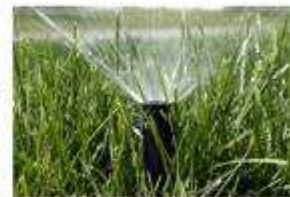
Reuse water can be used to irrigate baseball fields
