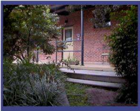
Courtyard Wastewater Treatment System at Triangle Business Park
