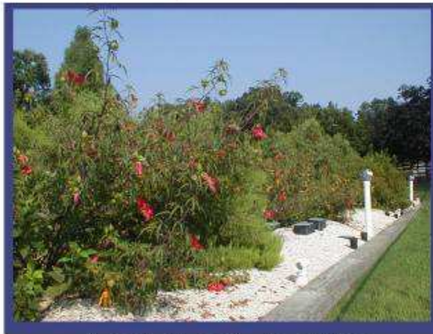
Vegetated Sand Filter at Chatham Central High School
