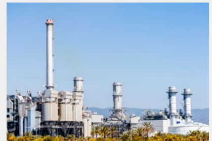
Serving as transaction advisor for a waste and recycling center PPP in the Middle East
