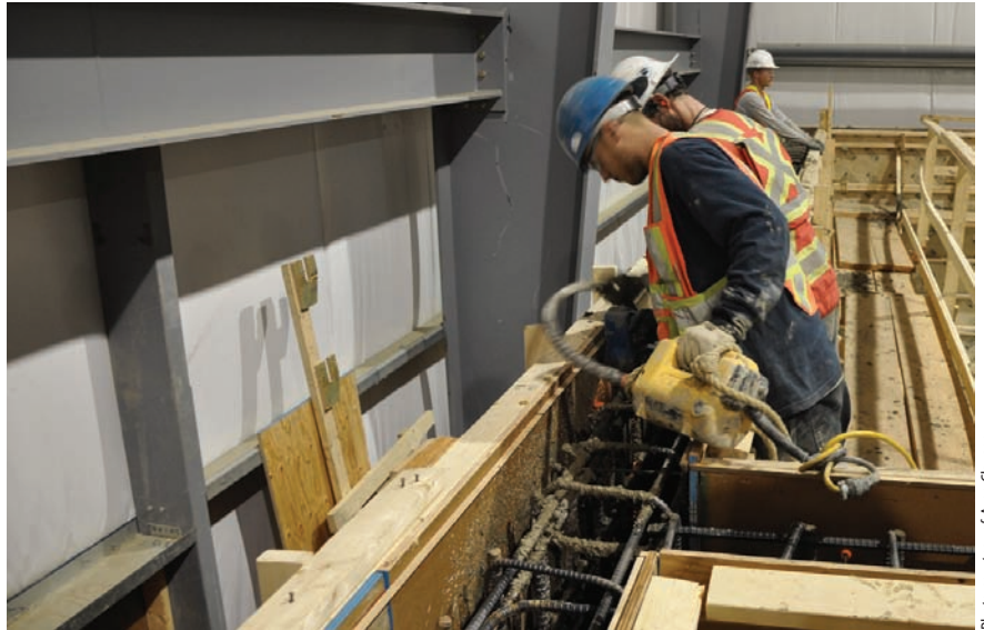
Vibrating the concrete in the mill building
