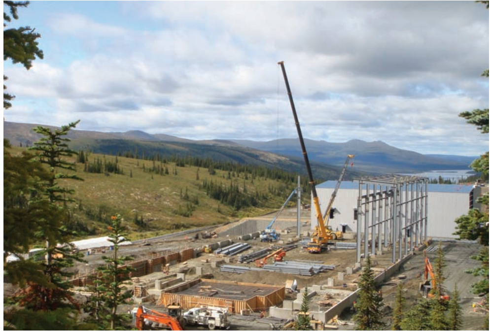
Construction underway on concentrate building
