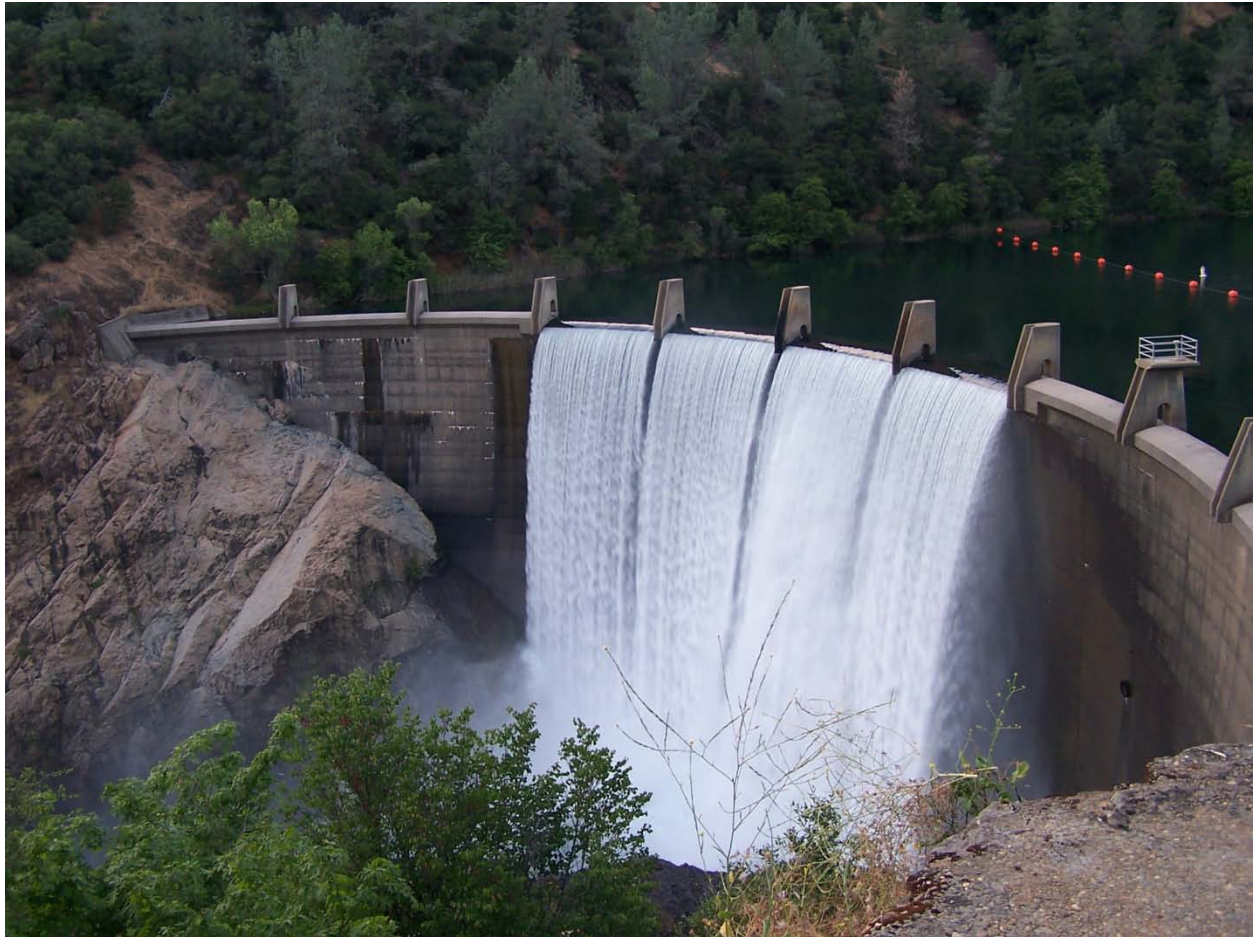
Figure 2. Flow Over North Fork Dam Spillway
