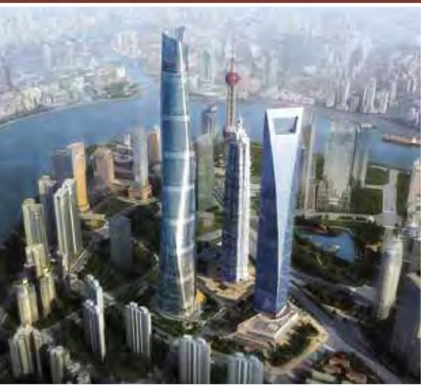
Tetra Tech is providing all the high performance building systems solutions and smart building technology for the 121-story Shanghai Tower
